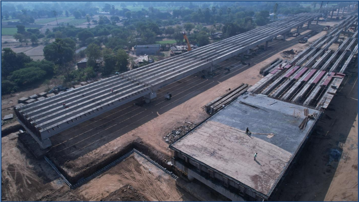
Work In Progress at Major Bridge ch. 352+281 A1 Side (Deck Slab)
