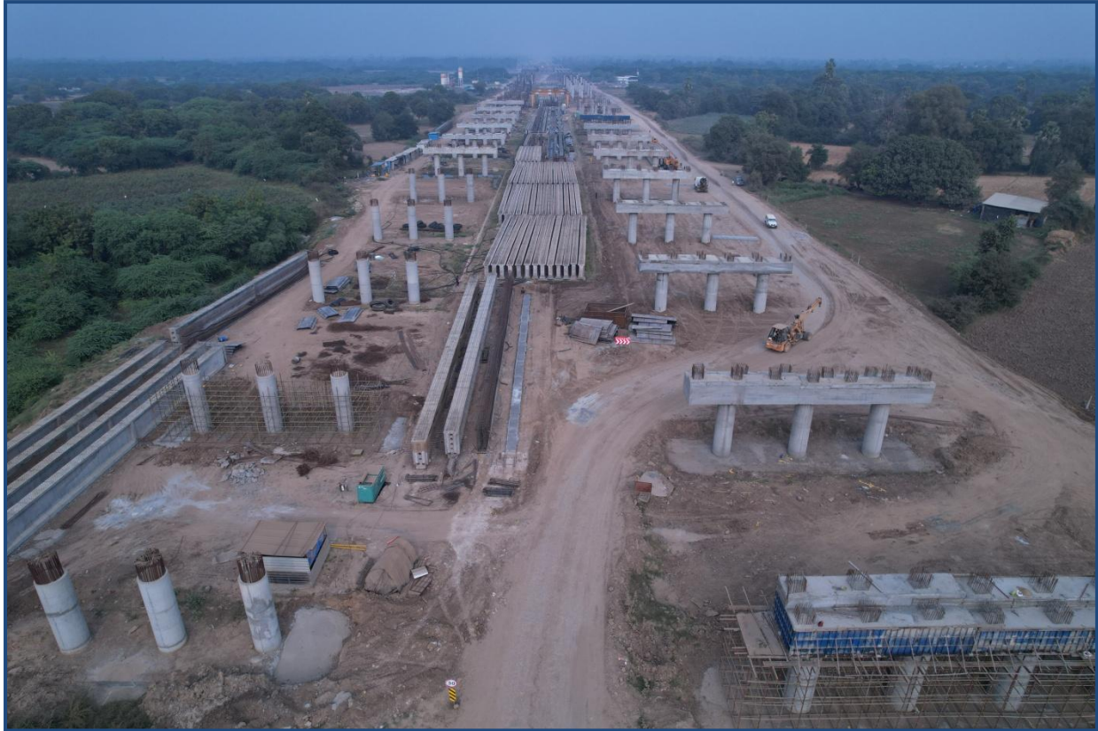
Work In Progress at Major Bridge ch. 352+281 A2 Side
