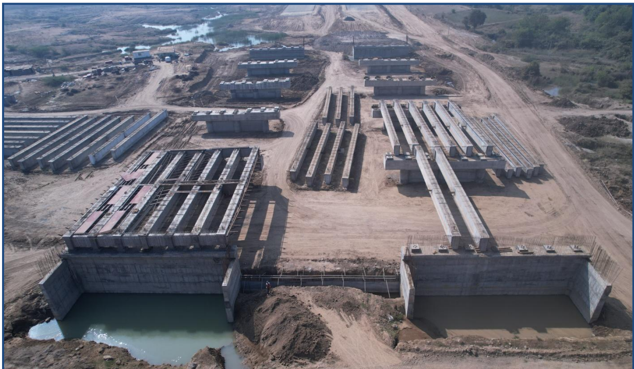
Girder launching at Major Bridge Ch-359+936
