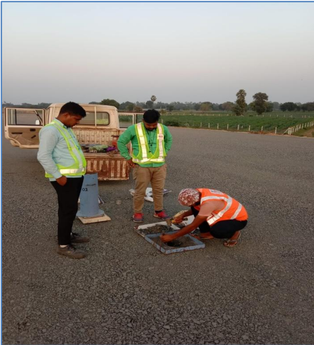
FDD checking at Ch. 351+150 GSB Top
